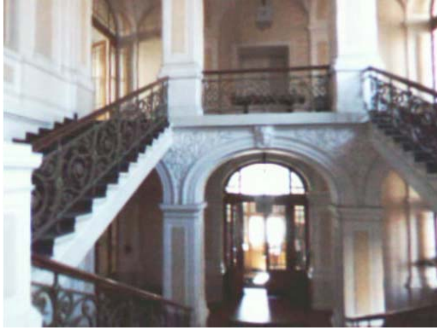
Figure 5: a view of the stairwell
